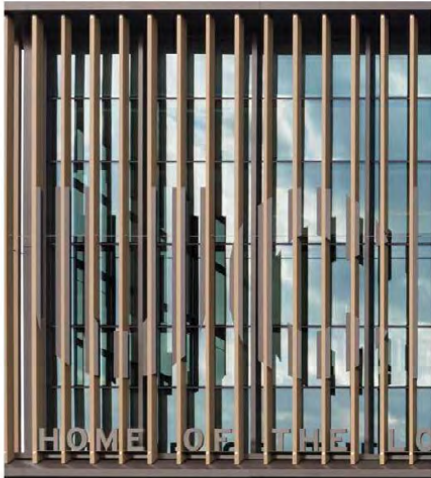
PPC aluminium vertical fins • Contemporary reference of traditional ornamentation
