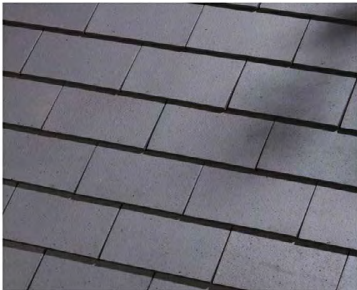
Rosemary clay tiled roof • Enhances area and references traditional materials • High quality and aesthetically pleasing
