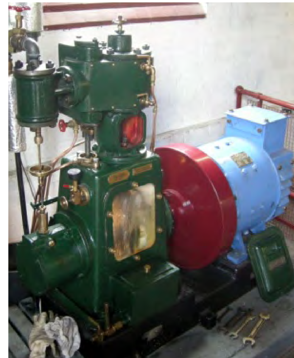
Reader steam engine driving GEC generator at Coleham Pumping Station (Courtesy gracesguide.co.uk).
